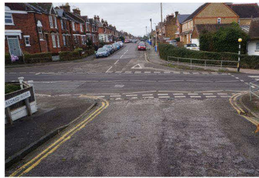
Aldred Road junction missing tactile and dropped kerb information
