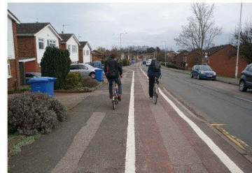
Shared walking and cycling facilities can reduce the comfort of walking routes
