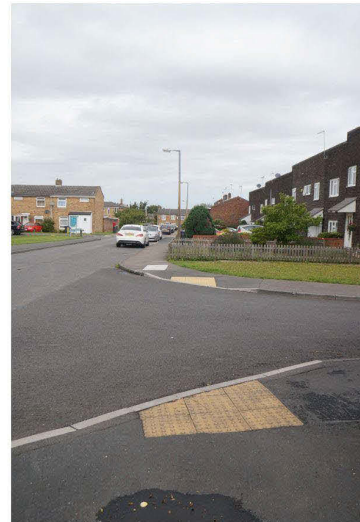
Misaligned crossing points pedestrians in direction of traffic
