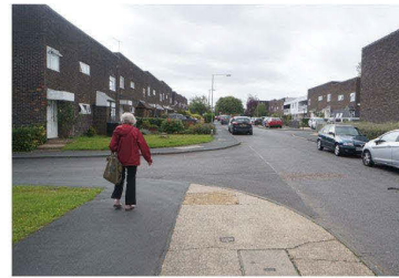
Example of junction missing both tactile paving and dropped kerbs
