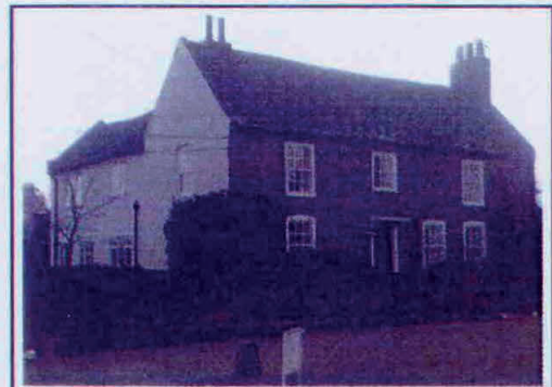
Figure 2- Hook Place farmhouse
