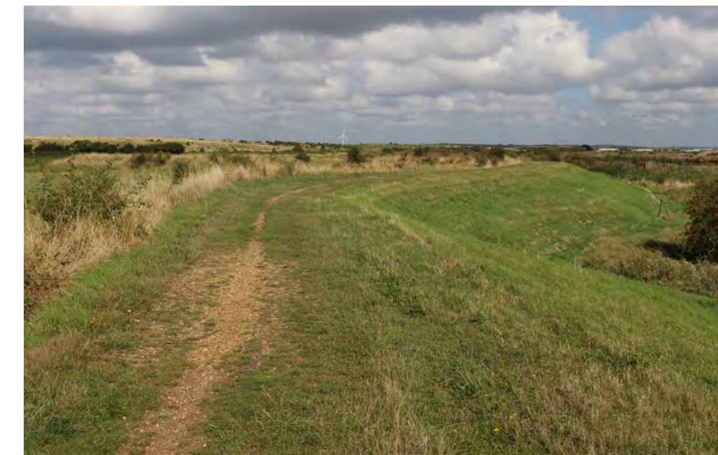
Figure 42. Site photo existing Dartford Marsh embankment
