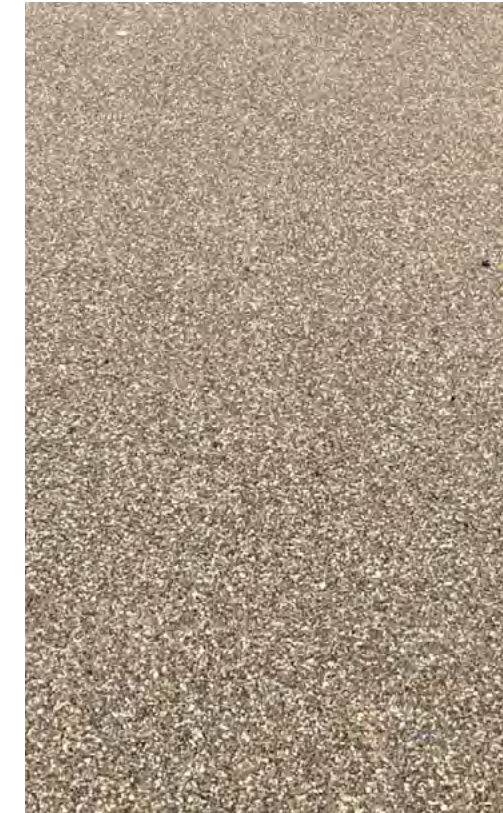
Figure 87. Buff coloured tarmac for roadways through new developments
