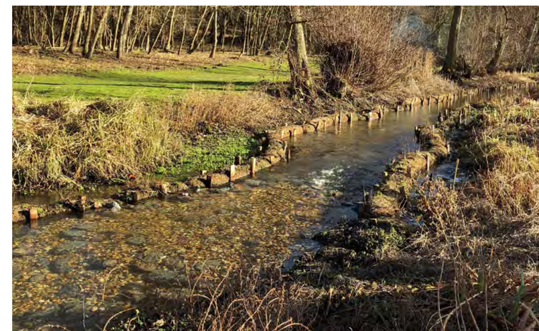
Figure 78. Brushwood mattresses restore river edge
