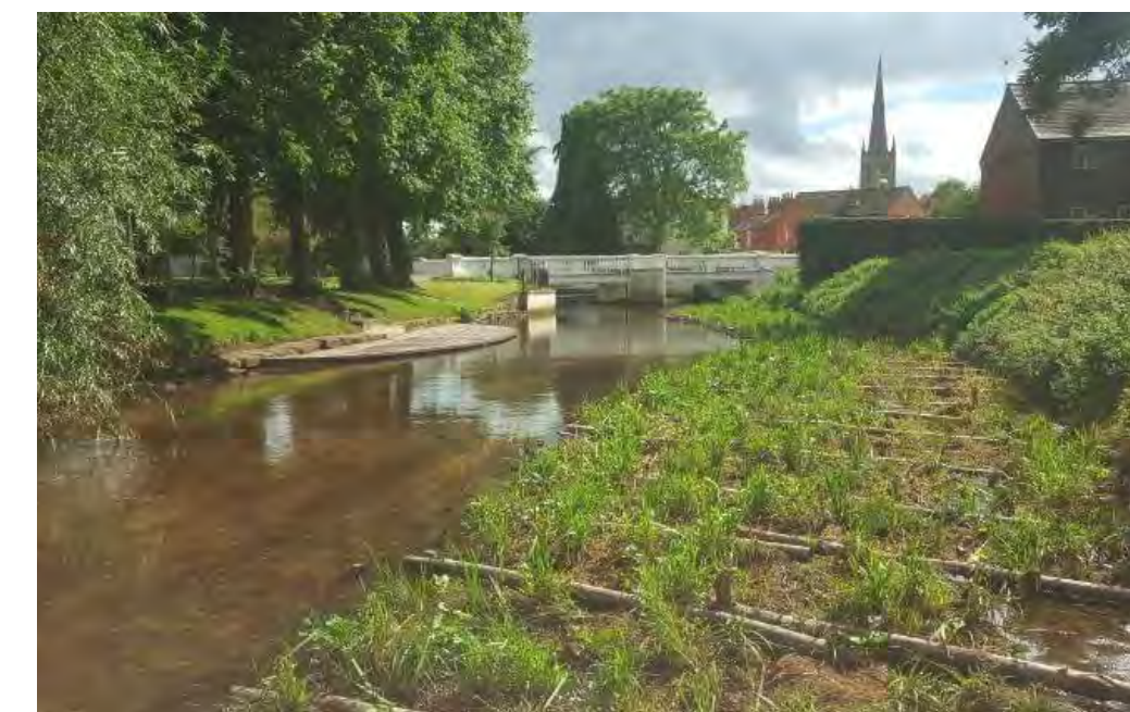
Figure 79. Angle of slope decreased using brushwood mattresses
