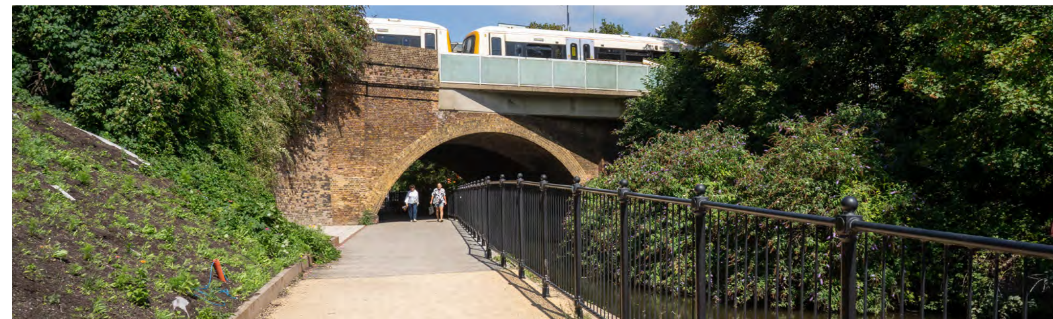
Figure 61. Existing black metal railings
