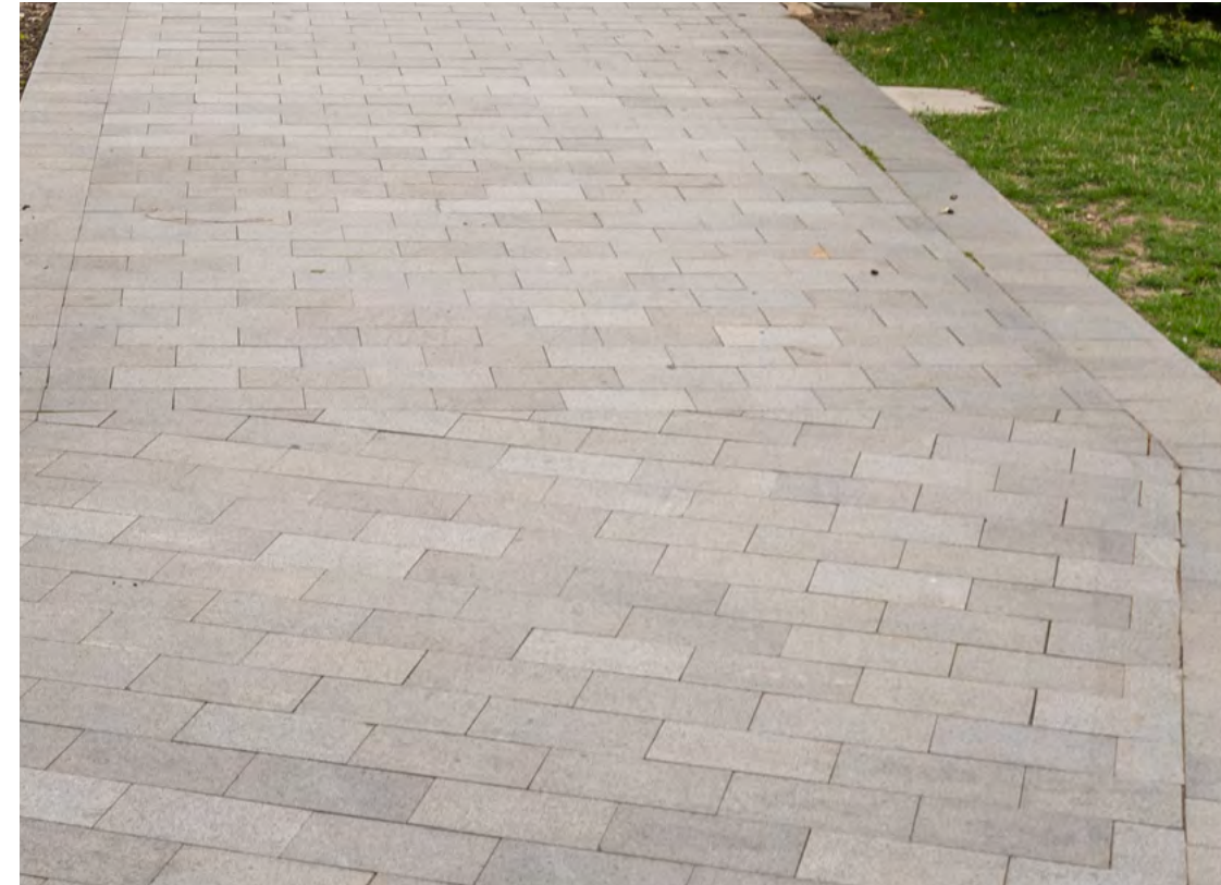
Figure 86. Porous Granite for public realm next to the River Darent 300 x 100mm
