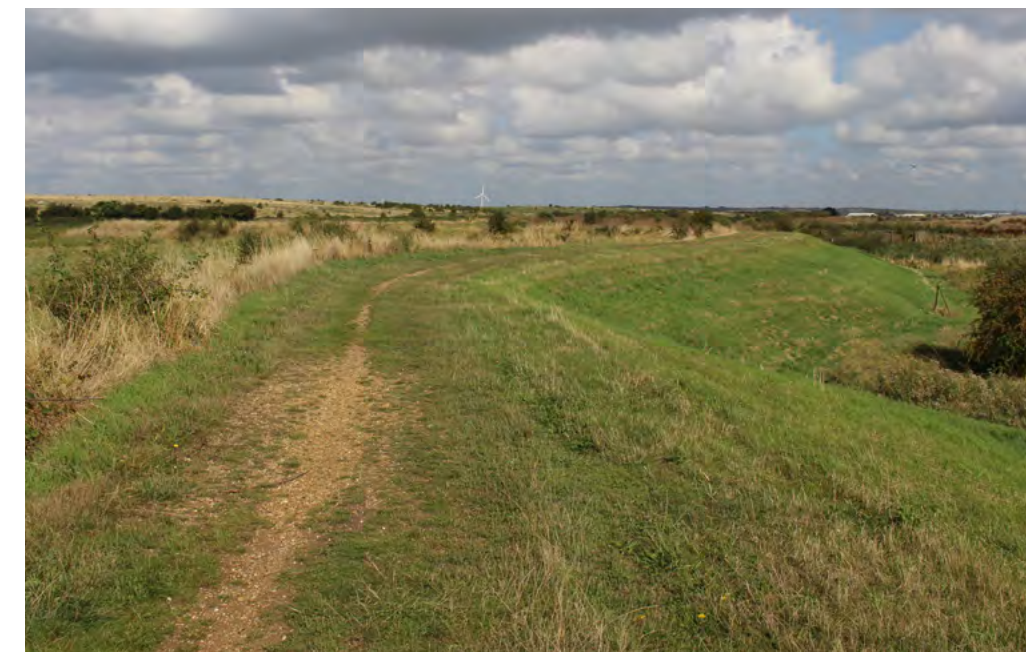
Figure 42. Site photo existing Dartford Marsh embankment
