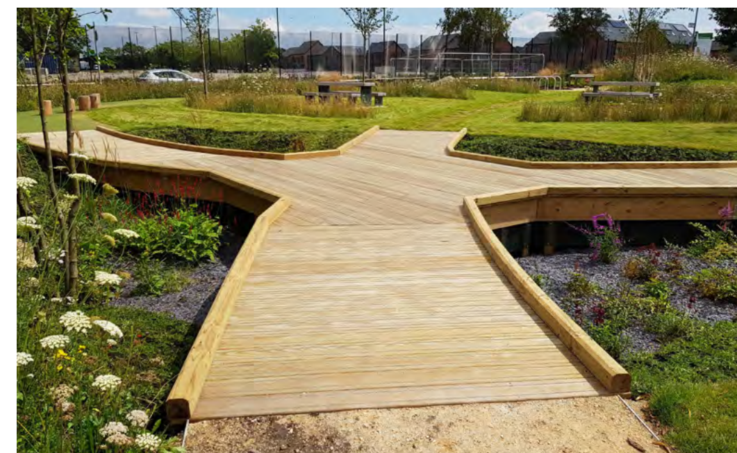
Figure 74. Timber boardwalk over a gravel planted attenuation basin
