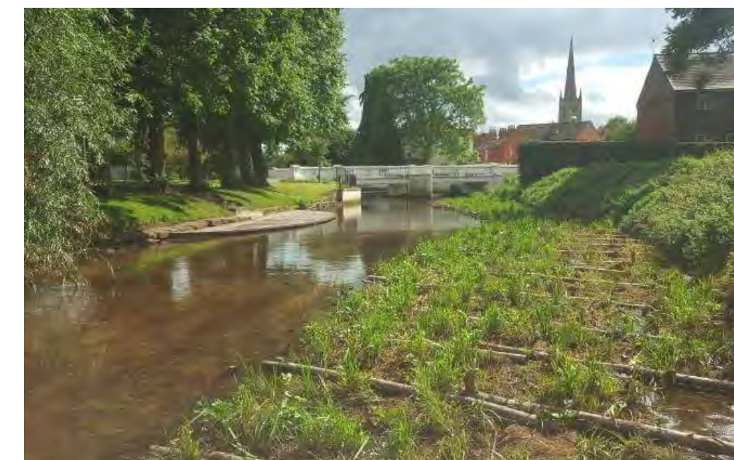
Figure 79. Angle of slope decreased using brushwood mattresses
