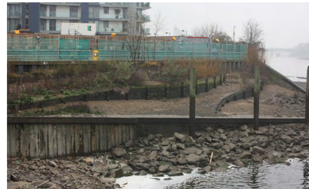
Figure 53. Cut down wall with installed terracing
