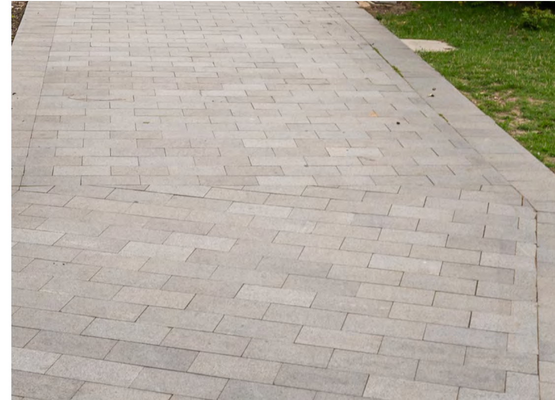
Figure 86. Porous Granite for public realm next to the River Darent 300 x 100mm
