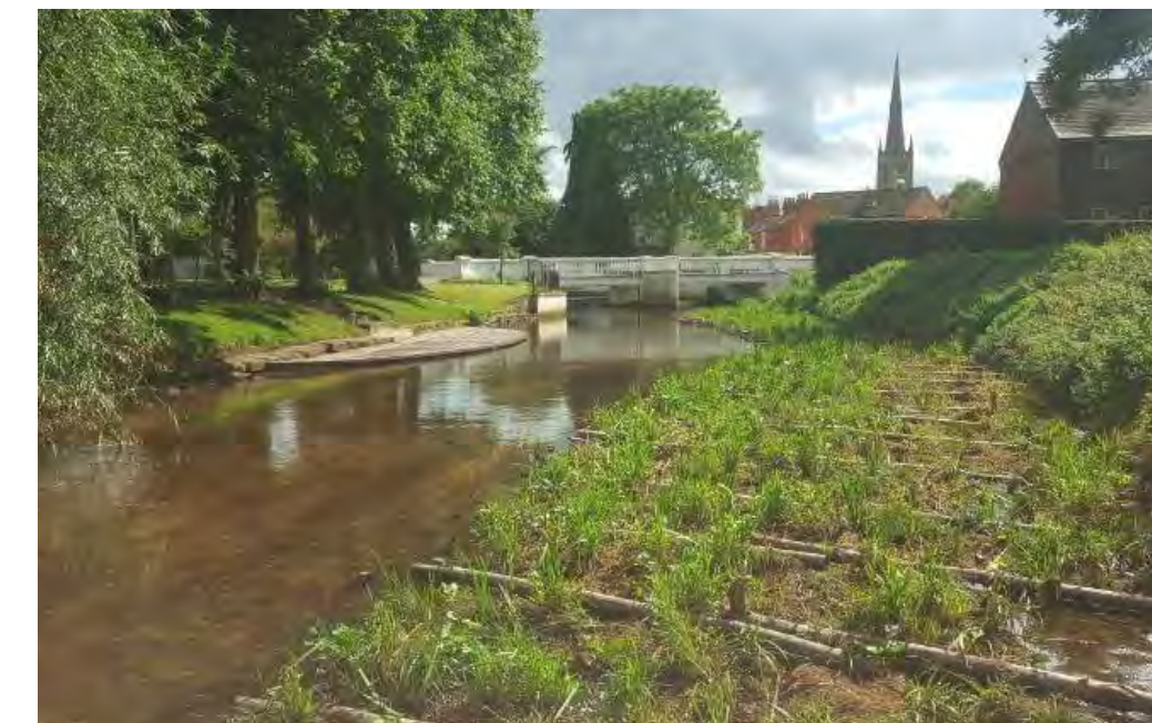
Figure 79. Angle of slope decreased using brushwood mattresses
