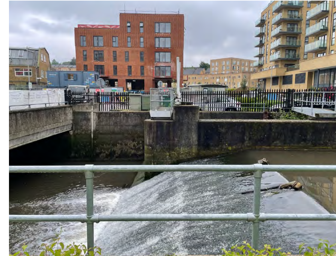
Figure 65. Site photo of the Wellcome Sluice
