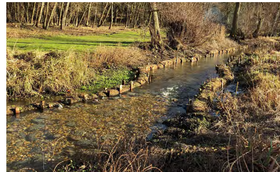
Figure 78. Brushwood mattresses restore river edge
