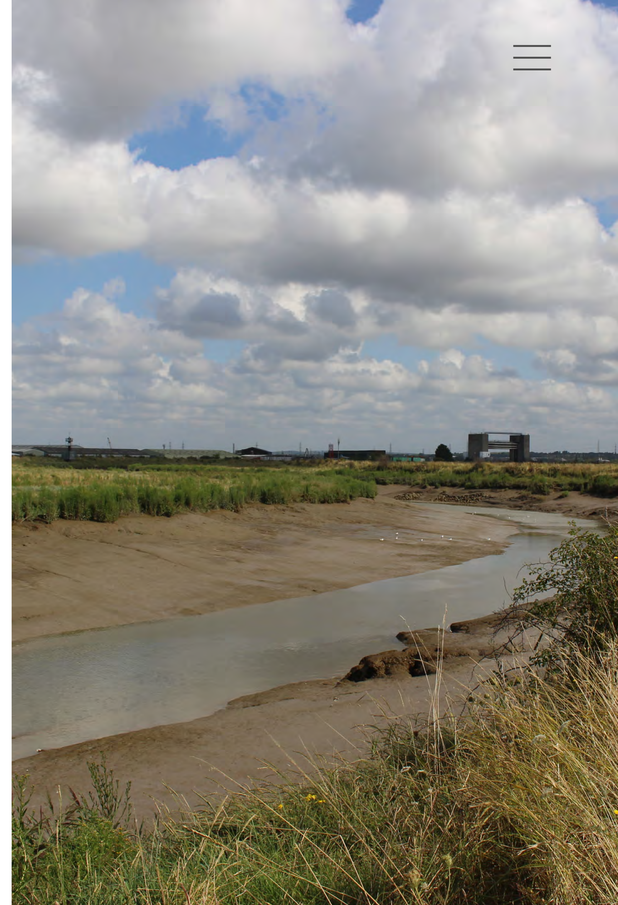
Figure 30. Site photo of the River Darent and Dartford Creek Barrier in the distance
