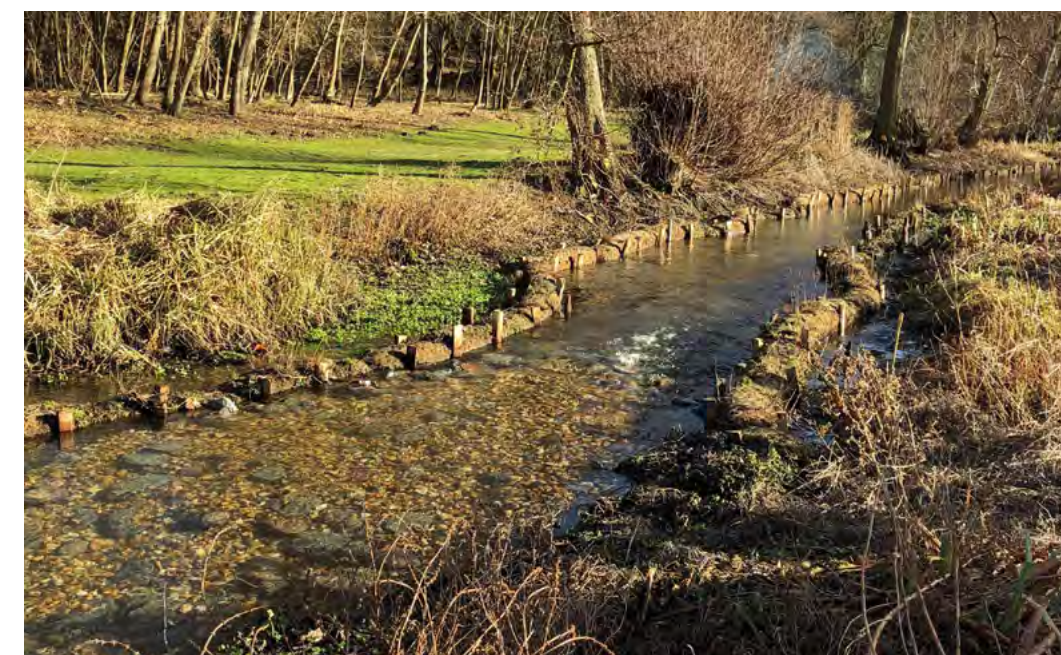
Figure 78. Brushwood mattresses restore river edge
