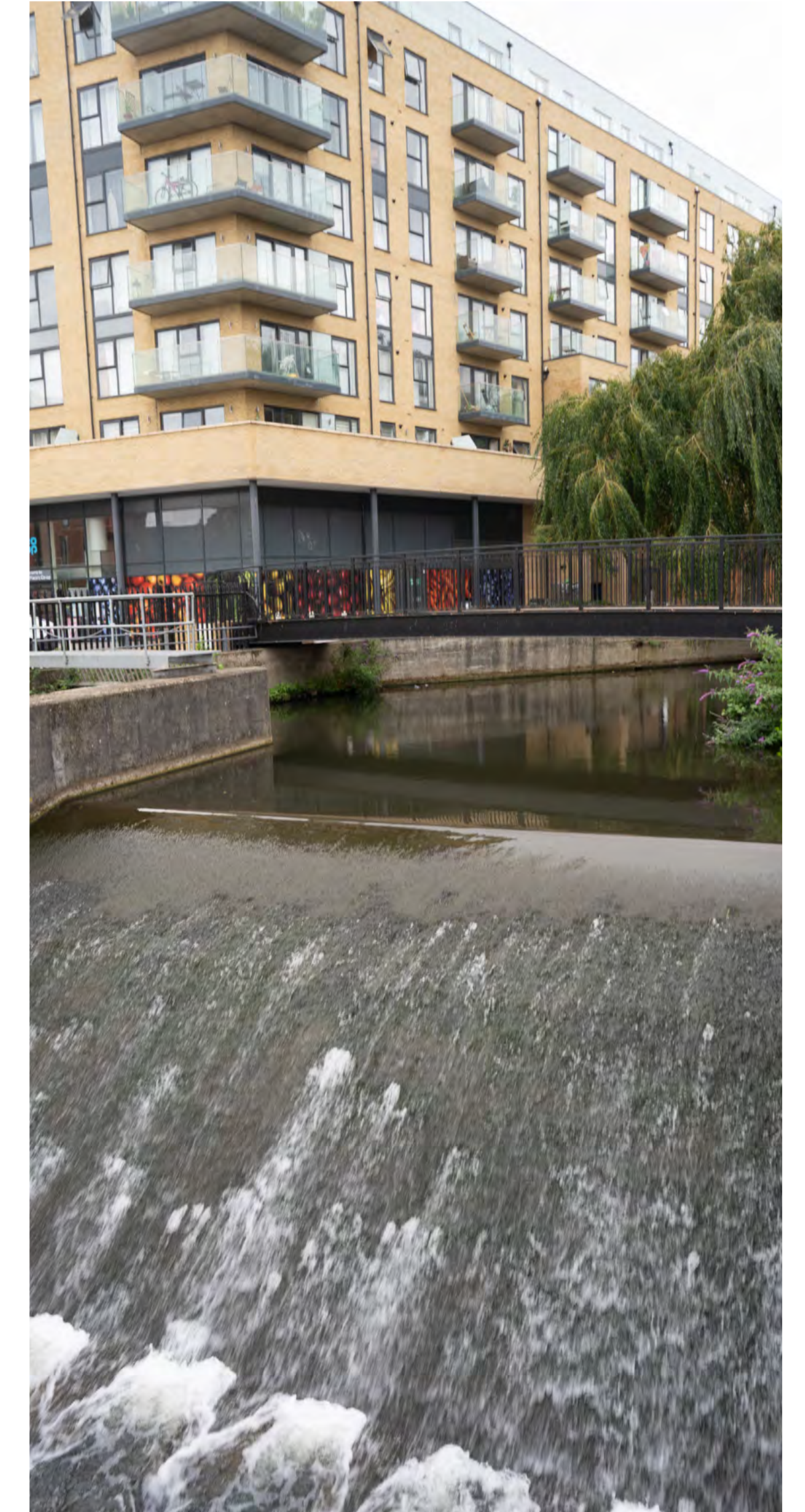
Figure 67. Site photo of the Wellcome Sluice
