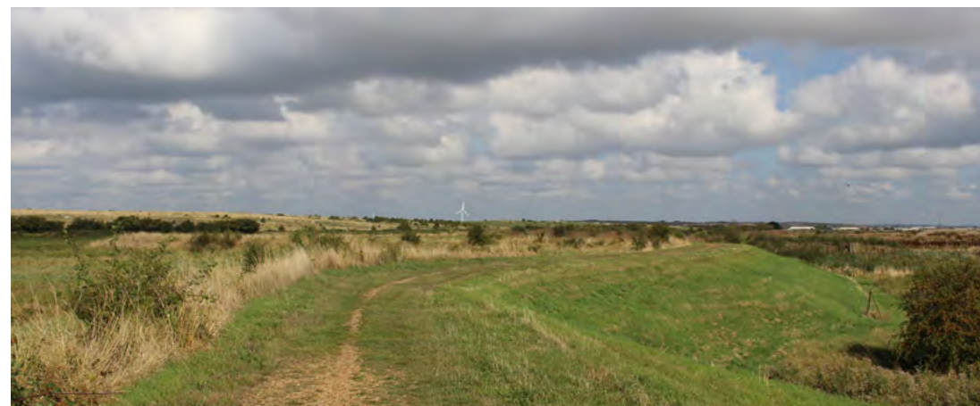
Figure 23. Existing embankment in Dartford Marshes
