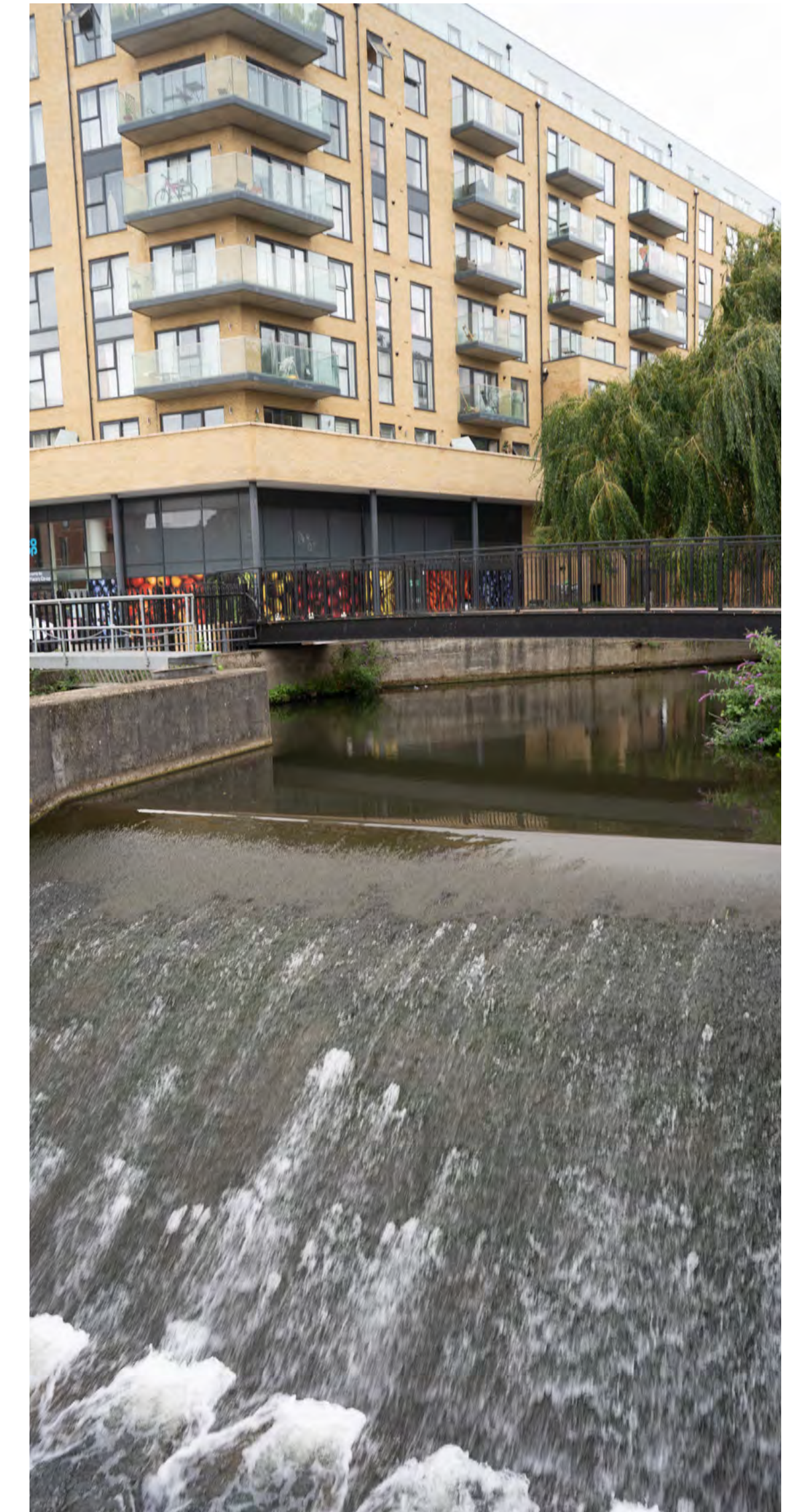
Figure 67. Site photo of the Wellcome Sluice
