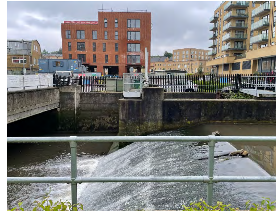
Figure 65. Site photo of the Wellcome Sluice
