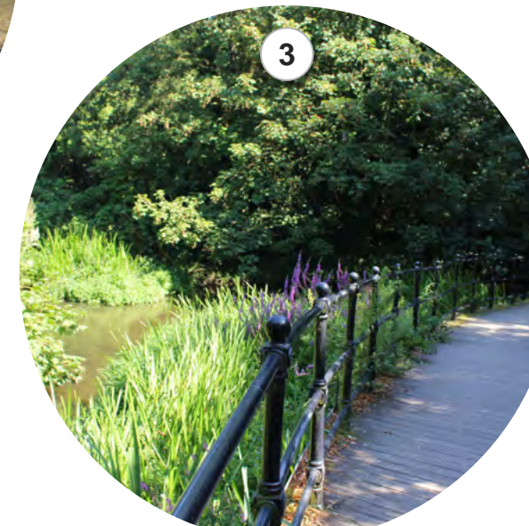
3. Timber deck edge to river
